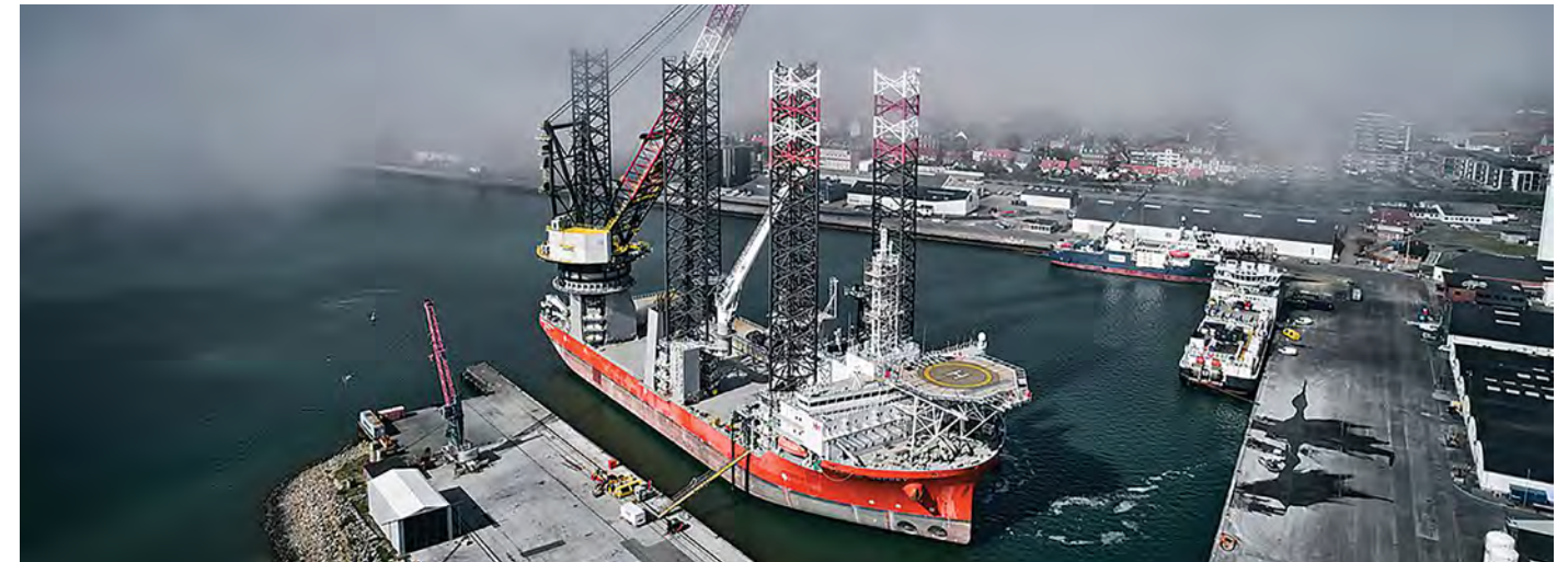
(Above) Pacific Osprey with new crane boom in the Port of Esbjerg.
